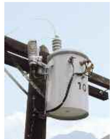
Single hanger bracket one high-voltage bushing self protected unit.
