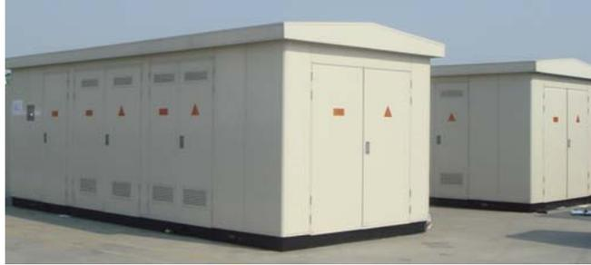
Fig. 7 Containerized Substations
