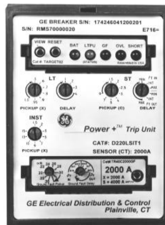
Figure 9. Power+™ Trip Unit.
