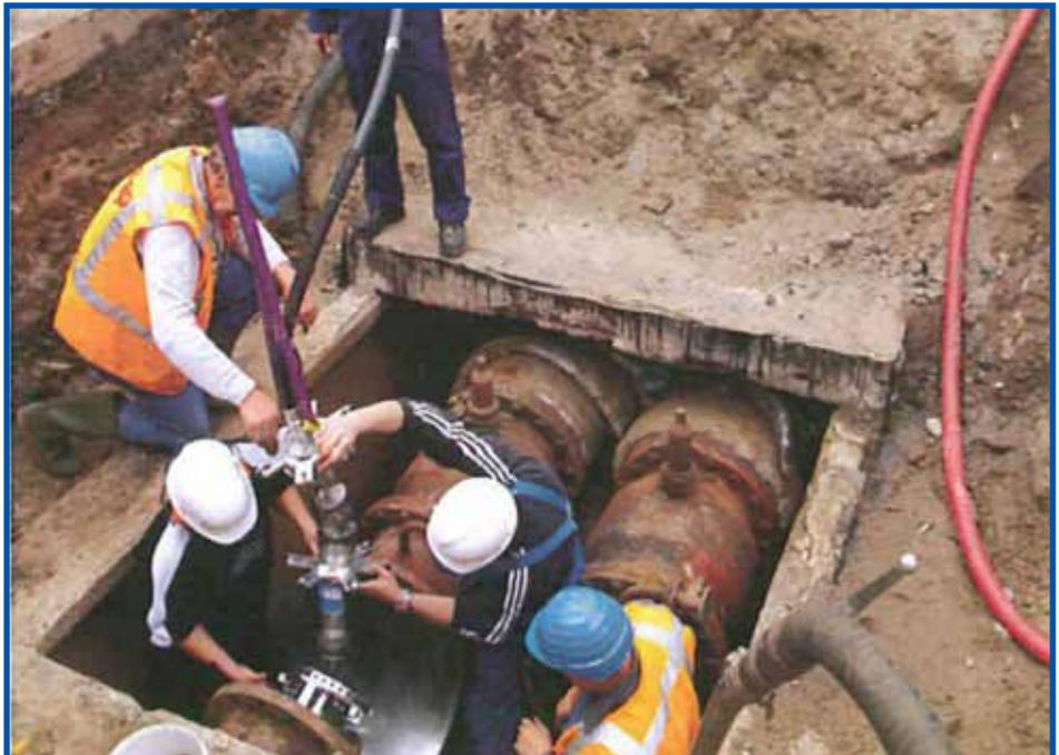
Figure 1. Tool inserted at removed valve.
