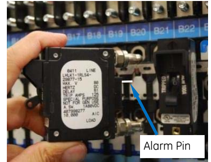
Correct Breaker orientation for insertion
