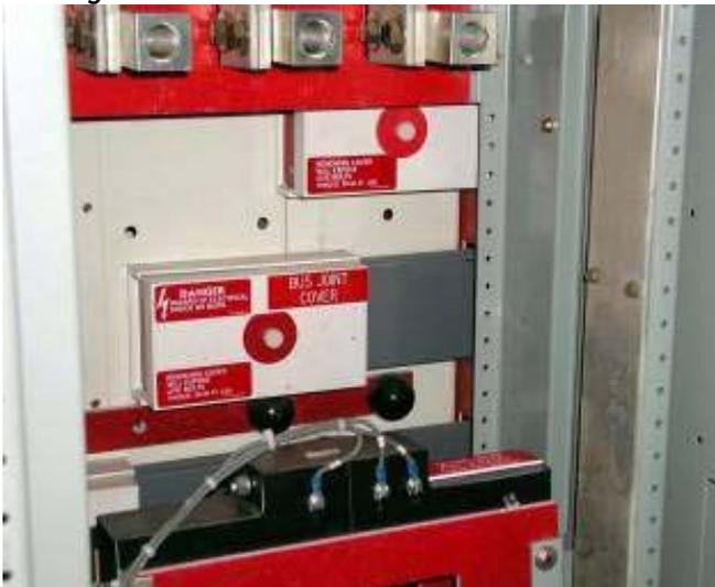
area is much safer to work around with the covers open. This option also drastically reduces the probability that a bus fault can happen.
