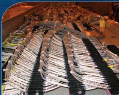
Above: Traditional switchgear wiring. Right: Entellisys' greatly reduced wiring means many fewer terminations and faster, easier installations.
