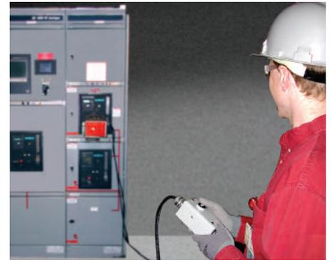
Arc-resistant medium-voltage switchgear (5kV to 38kV) directs and controls arc flash energy to minimize injury to personnel and reduce damage to surrounding equipment. Additional features include:
