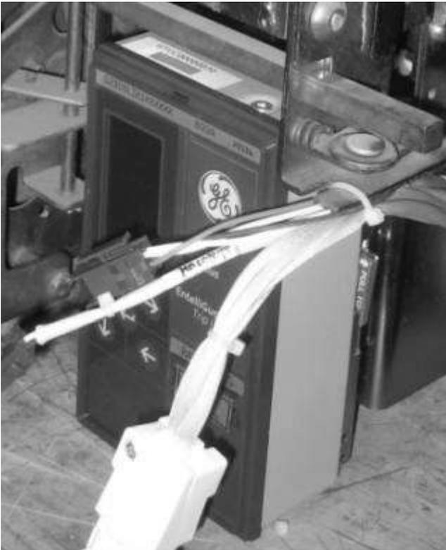
Figure 26. Trip unit installed on the breaker (RL-1600 shown)
