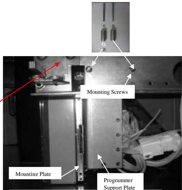
Figure 17: Mounting plate and support bracket mounted on the breaker
