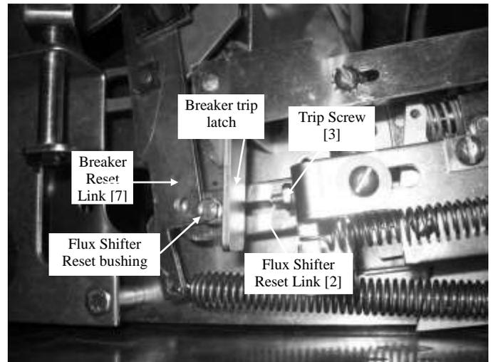
Figure 5b. Flux shifter assembly installed, as viewed from the side of the breaker (RL-3200/4000 shown).
