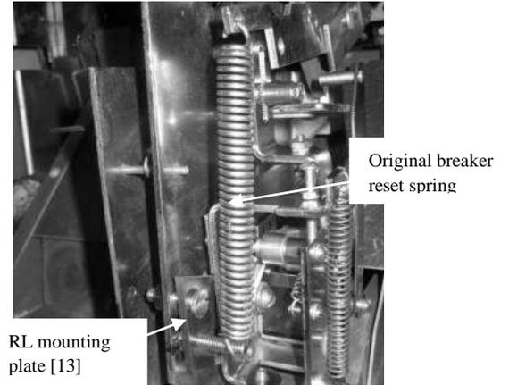
Figure 5a. Flux shifter assembly installed, as viewed from the side of the breaker (RL-1600 shown).
