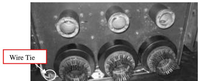
Figure 20: Installing the CTs on an RL-3200 breaker
