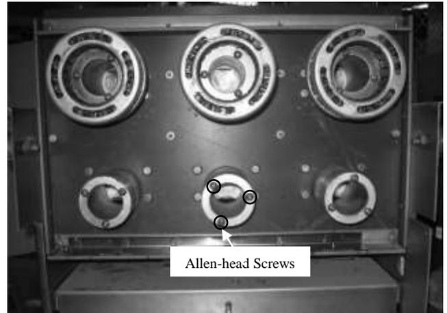
*Figure 1: Primary disconnects removed from bottom studs*
