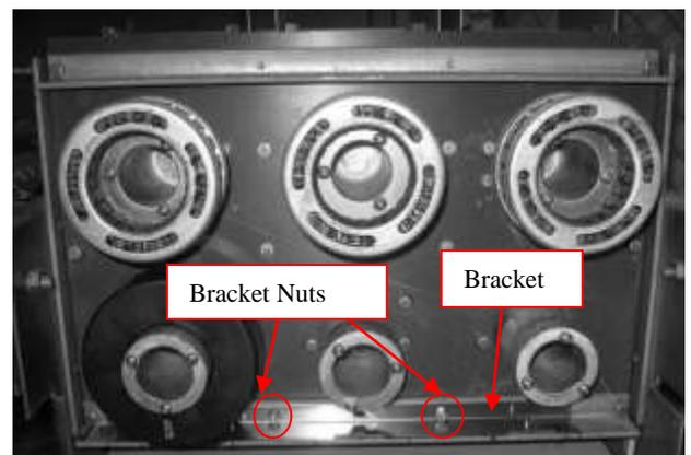
Figure 23: Installing the CTs on an LA-3000 breaker
