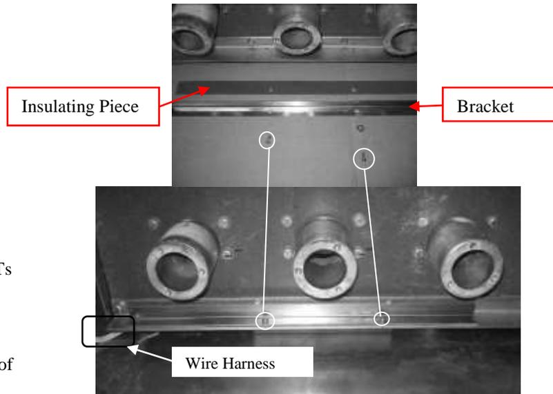
Figure 19: Attaching bracket and insulating piece to breaker bracket (RL-3200 shown)
