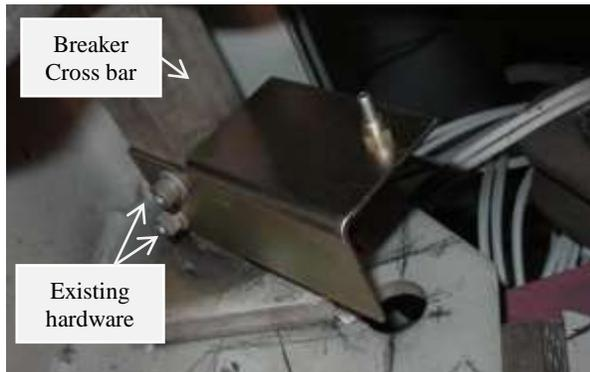
Figure 4: Installed Reset Assembly
