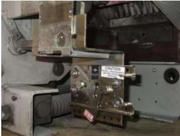
*Figure 14: Trip Unit bracket mounting*
