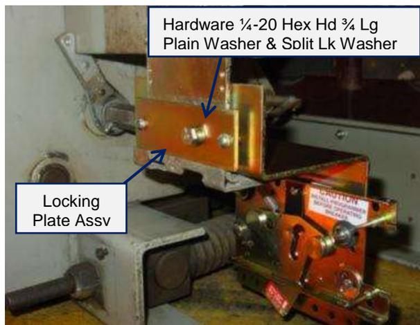
*Figure 15: Securing Trip Unit bracket*
