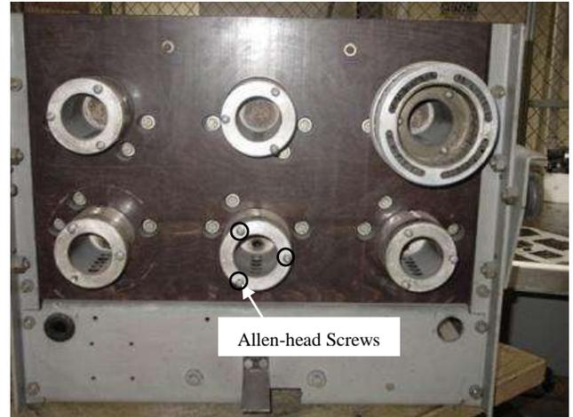
*Figure 1: Primary disconnects removed from bottom studs*
