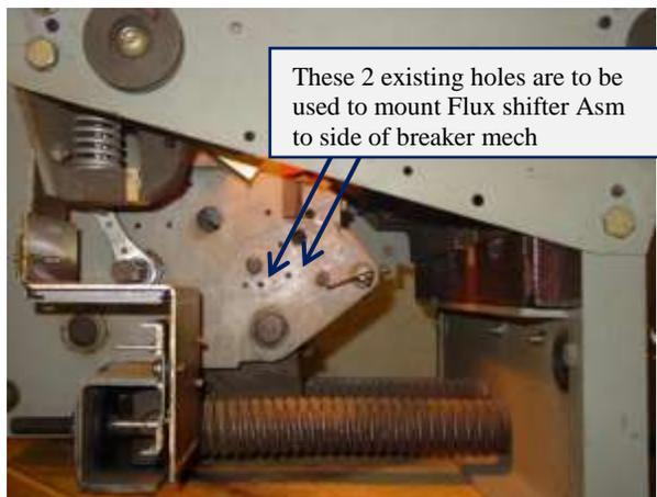
Figure 5: Flux Shifter mounting location
