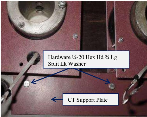
Figure 17: Installing Current sensors
