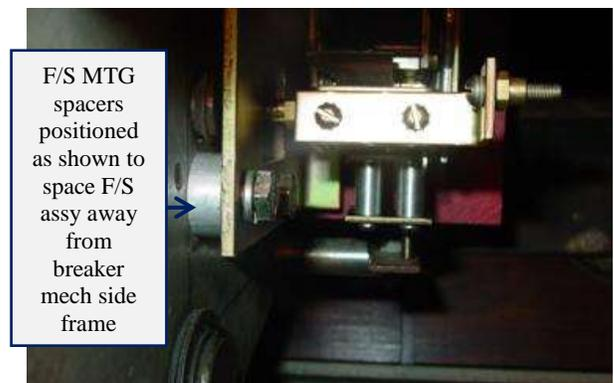
Figure 7: Flux Shifter mounting
