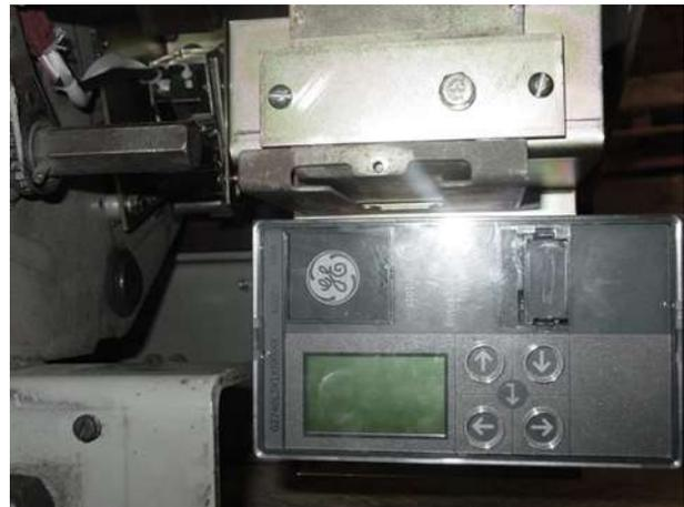
Figure 20. Trip unit installed on the breaker
