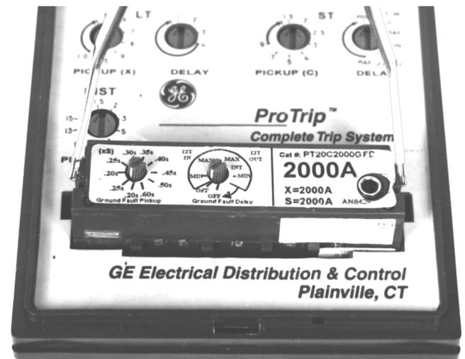
Figure 13. Removing the interchangeable rating plug.
