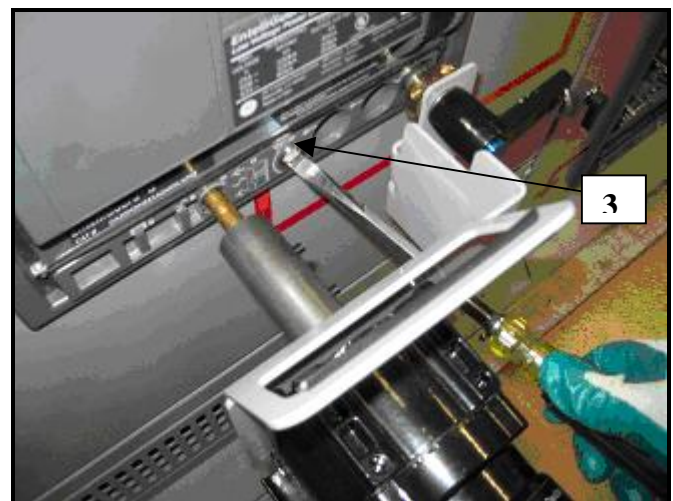
Fig. 3 Opening Racker access door
