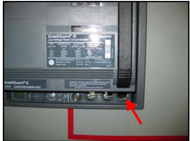
Fig. 1 Remote Racking Operator mounting Port.
