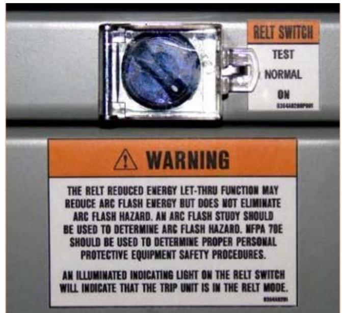
Figure - 3: Three-position lockable RELT control switch with built-in indicating light.
