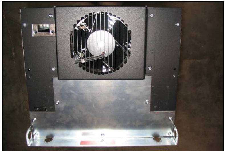
Figure 3. Top cover plate installed
