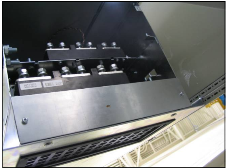
Figure 12. Bottom air inlet cover installed
