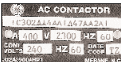
Figure 1. High-Voltage Contactor Nameplate
