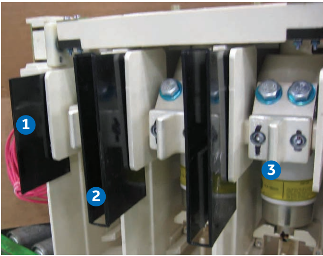
Figure 11. 400A Stab-In Contactor Parts
