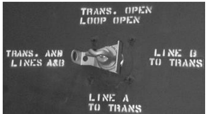
Figure 26. V-blade switch.
