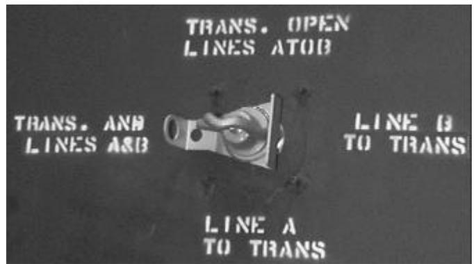
Figure 25. T-blade sectionalizing switch.
