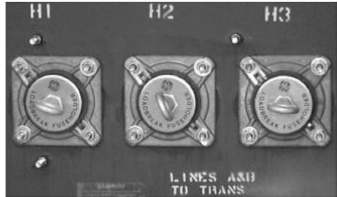
Figure 9. Loadbreak fuses.
