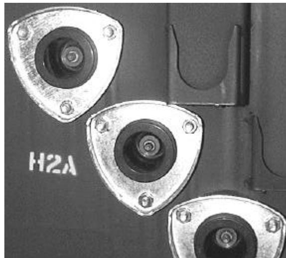
Figure 13. Separable insulated connectors (typical arrangement)..
