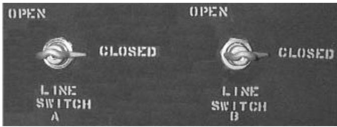
Figure 18. Loop-feed switches.
