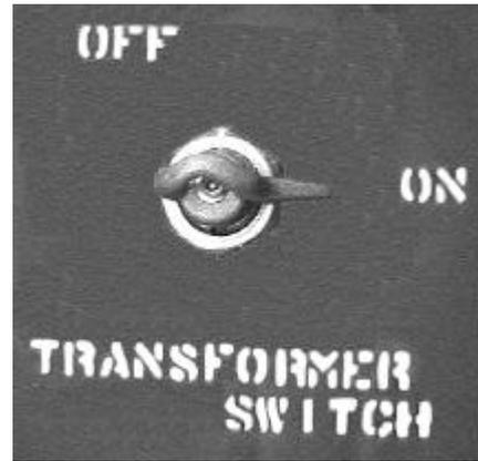
Figure 16. Radial-feed switch.
